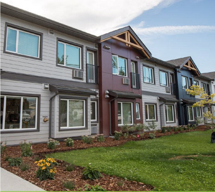
KIKÉKYELC in Kamloops, built to BC Energy Step Code Level 3 and opened in September 2020.
