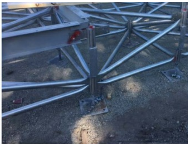
Steel-web foundation in 137 E 37th Avenue, Vancouver modular project.
