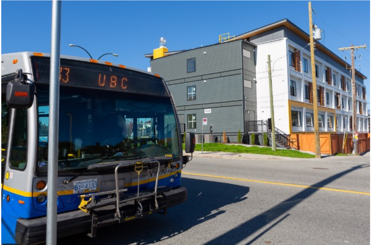
Three Storey 52 units modular Sarah Ross Housing at 4480 Kaslo Street, Vancouver - Transit close by the property.
