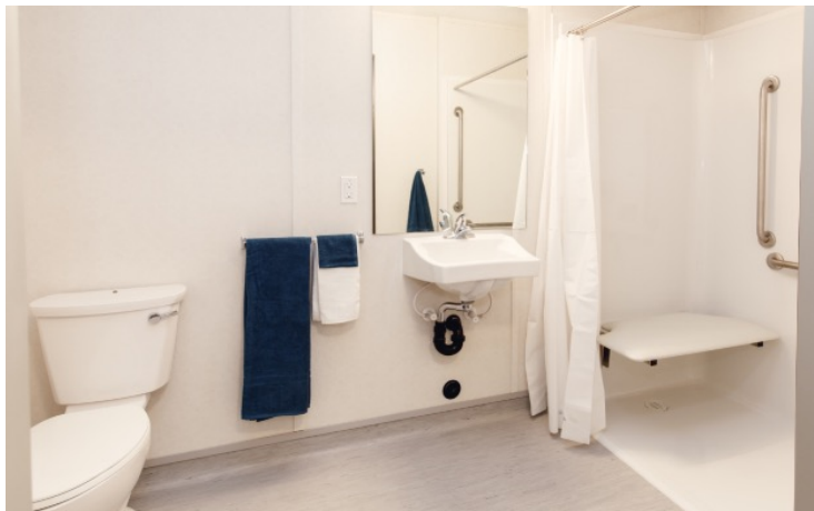
Wheelchair accessible washroom
