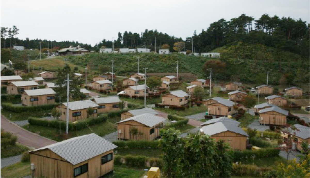
Temporary Lodging - single family RV park complex - Rikuzentakata, Iwate Prefecture, Japan.
