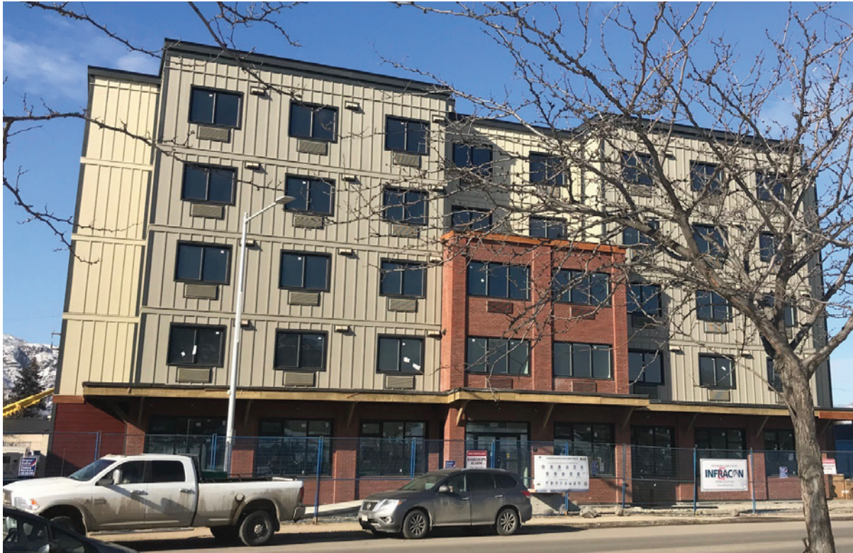
Five-storey modular housing at Tranquille Road in Kamloops.
