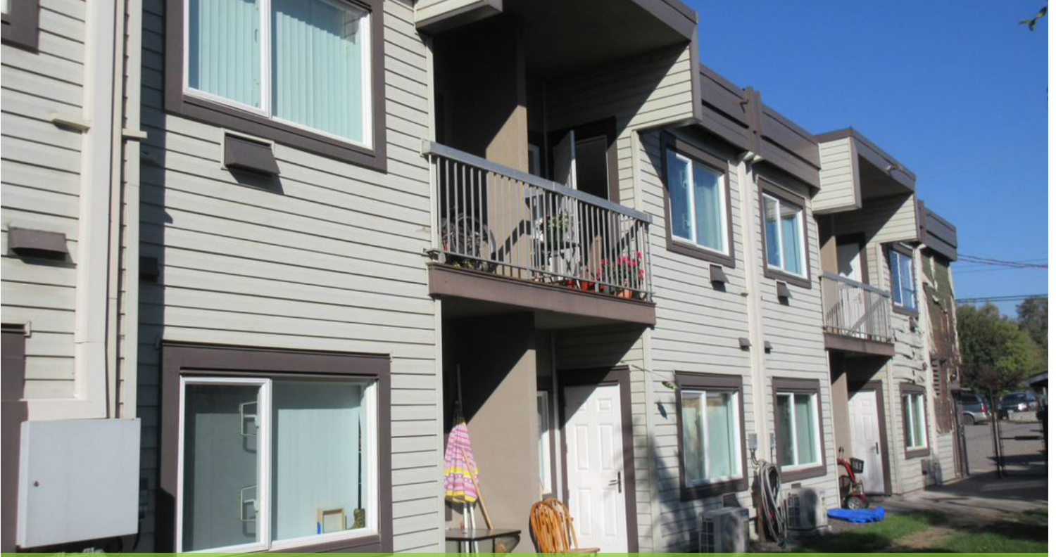
The Deep Energy Retrofit at Creekside Village in Vernon, B.C., achieved 81,300 kWh in energy savings.
