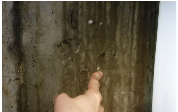
Figure 10.1 Investigation of moisture ingress should include a detailed review of the exterior assemblies, including at below-grade to above-grade transitions.
