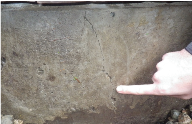
Figure 10.1 Investigation of moisture ingress should include a detailed review of the exterior assemblies, including at below-grade to above-grade transitions.
