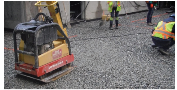
Figure 5.1 Example of clear crushed gravel placed and compacted for underslab drainage.
