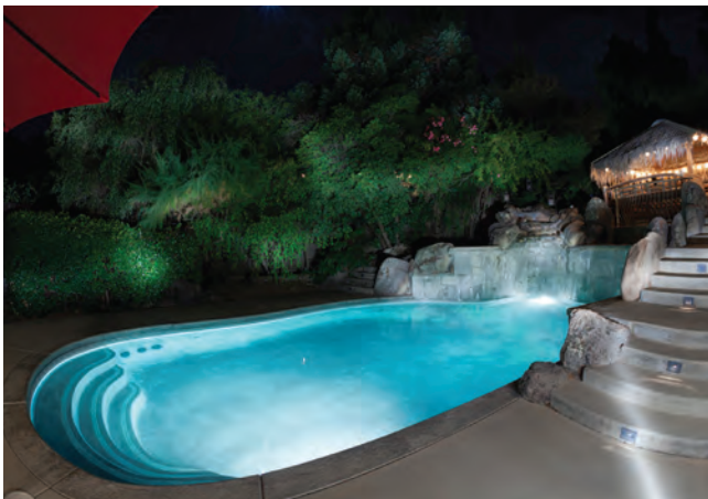
Good light levels in and around pools and hot tubs improves safety and security
