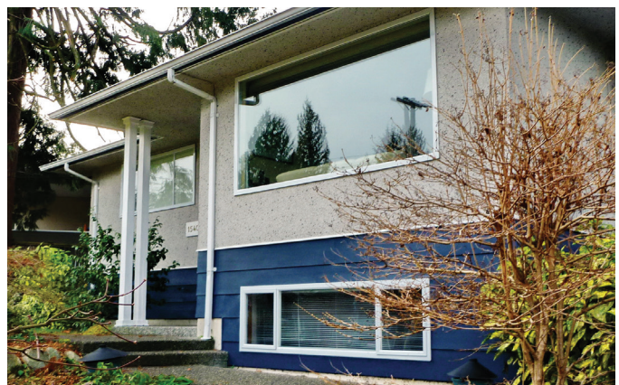
The upper windows on this home are protected by overhangs, allowing for more options when selecting products or evaluating installation methods.
