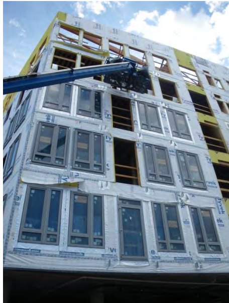
A 5+1 storey wood-frame MURB under construction in Portland, Oregon.
