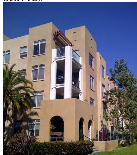
Californian style MURB Architecture in Southern California - While a face-seal stucco application may perform well in a hot and dry climate zone, in wetter climate zones the lack of overhang protection will result in the need for more robust wall assemblies and details (rainscreen).
