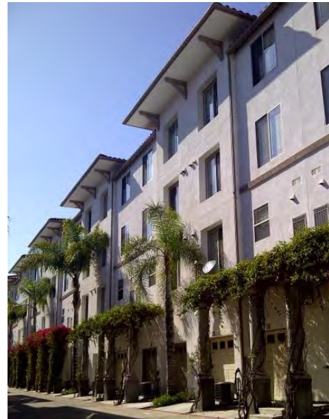
The roof overhangs of this MURB in Climate Zone 4 (hot) are an architectural feature that provides some solar shading to reduce solar heat gain through the upper-floor windows. Adjacent buildings will also shade some orientations of the building over the course of a day.
