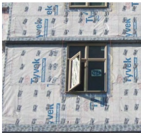
The use of cladding, such as masonry veneer, that relies on localized penetrations of the sheathing membrane by metal ties will increase the potential for tearing of air-barrier materials. The use of self-adhered membranes at brick ties helps reinforce these locations.
