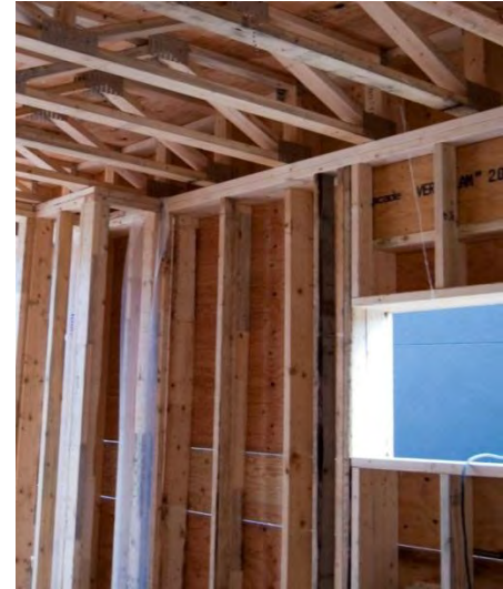
Pre-fabricated double-stud wall assembly. Photo courtesy: Winton Global Homes
