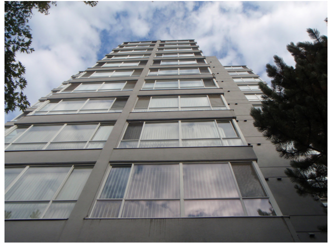
Figure 3 – Example of window wall glazing in a high-rise residential building
