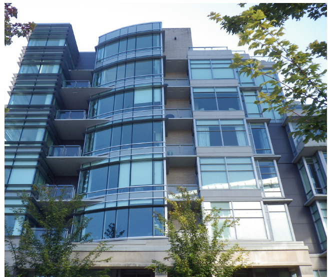
Figure 4 – Example of curtain wall glazing in a mid-rise residential building
