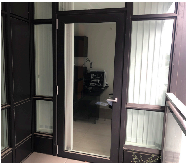
Figure 9 – Example of an aluminum frame swing door
