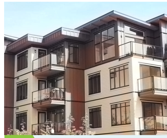
The upper deck is located over an enclosed space, while the balconies are not.
