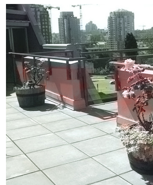
Deck with combination of guardwalls and guardrails.
