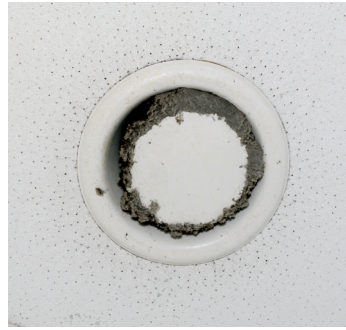
Condensation build up is caused by lint and dirt accumulation in ducts or vent covers and by restrictions in ducts.
