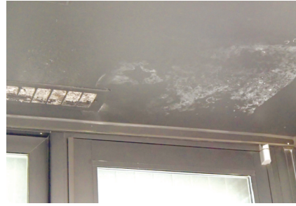
Poorly designed or unmaintained ducts can lead to damaged finishes from condensation build up.
