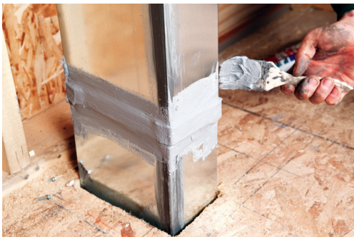
Duct sealing from the outside.
