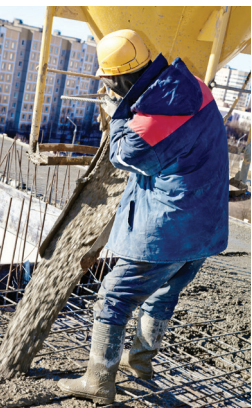
In-slab ducting cast into concrete during building construction.
