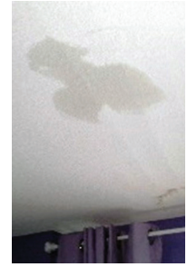
Poorly designed or unmaintained ducts can lead to damaged finishes from condensation build up.
