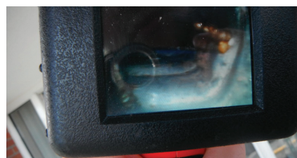
Scoped cameras provide views of duct interiors.
