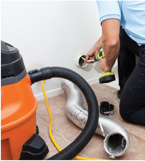
Condensation build up is caused by lint and dirt accumulation in ducts or vent covers and by restrictions in ducts.
