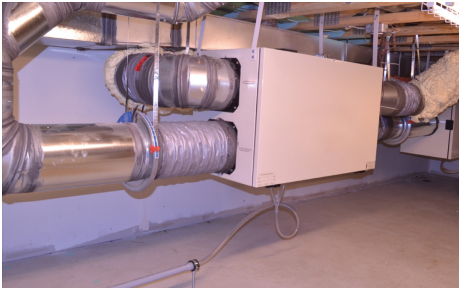
Figure 1: Example HRV System installed in a home.
