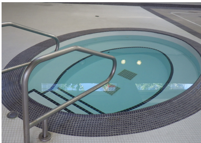
Example of a hot tub or “spa” in a residential building
