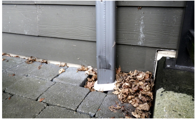
Example of a downspout leading to a perimeter drain
