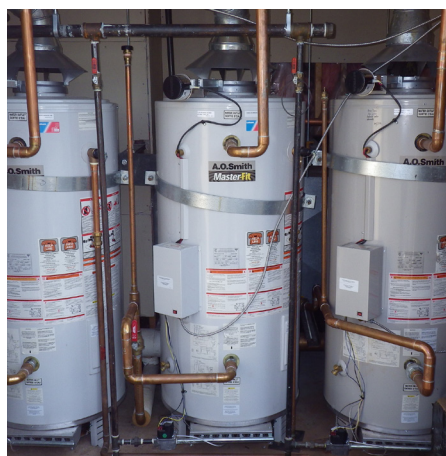
Example of natural gas fired water heaters for domestic hot water use
