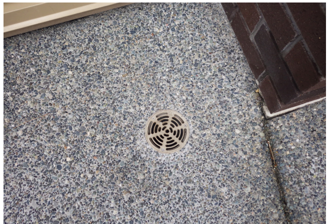
Example of a drain on a roof deck
