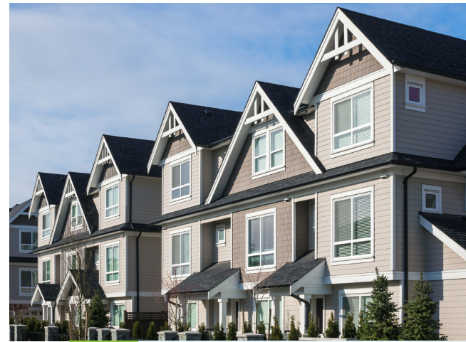
Lack of maintenance and replacement of aged or degraded sealants can cause damage to the building envelope and will negatively affect its durability.
