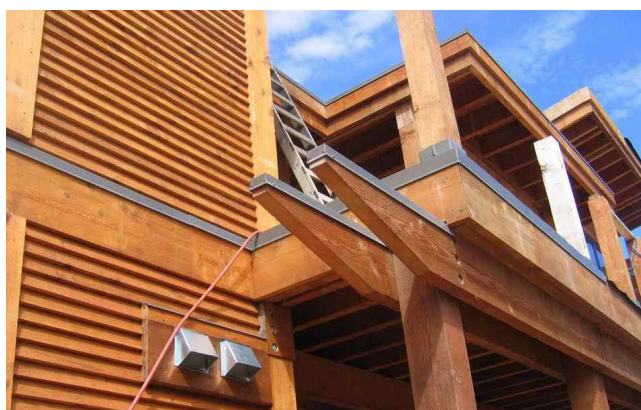
Metal cap flashing on exposed beam ends prevents water from collecting on the upper horizontal surfaces.
