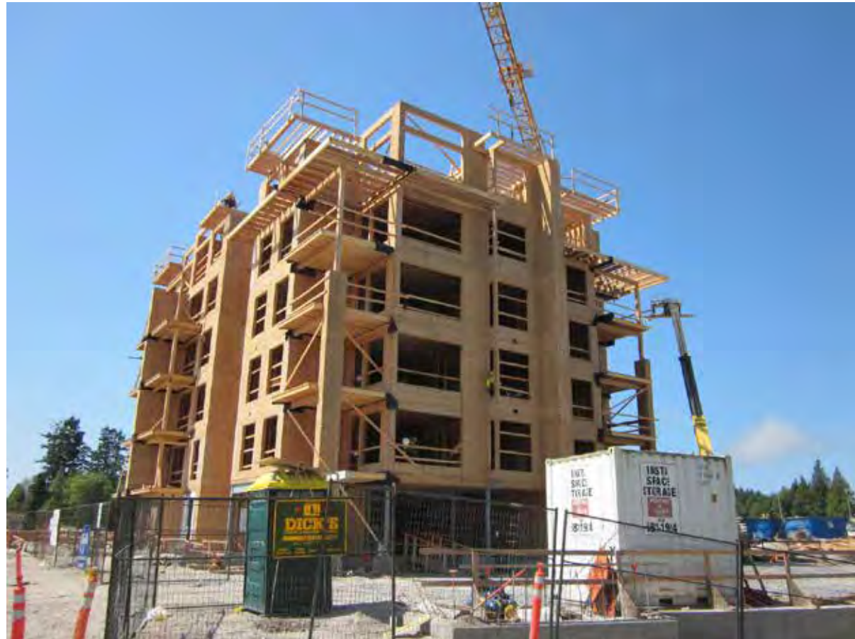
FIGURE 7.4 – SAIL: A CRANE WAS POSITIONED BETWEEN THE PHASE 1 AND PHASE 2 BUILDINGS
