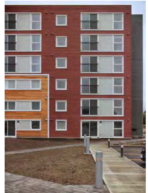
FIGURE 6.6 – HILLCREST VILLAGE: NO PROJECTING BALCONIES
