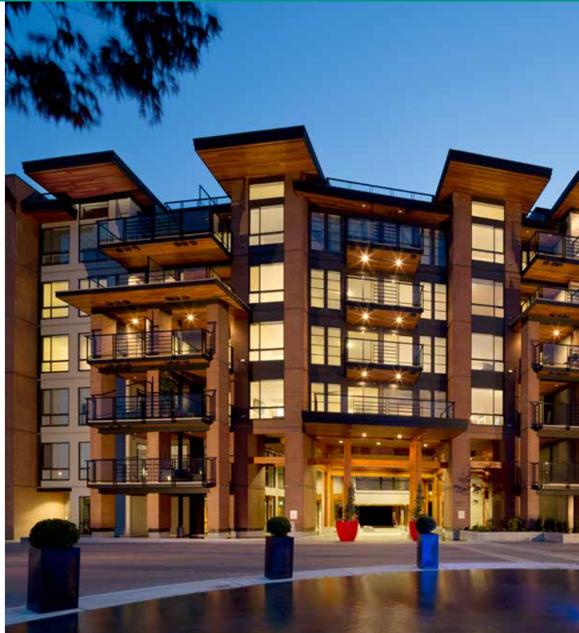
FIGURE 2.10 – THE SHORE IS A FOUR-PHASE MARKET CONDOMINIUM PROJECT LOCATED ADJACENT TO MOSQUITO CREEK IN NORTH VANCOUVER
