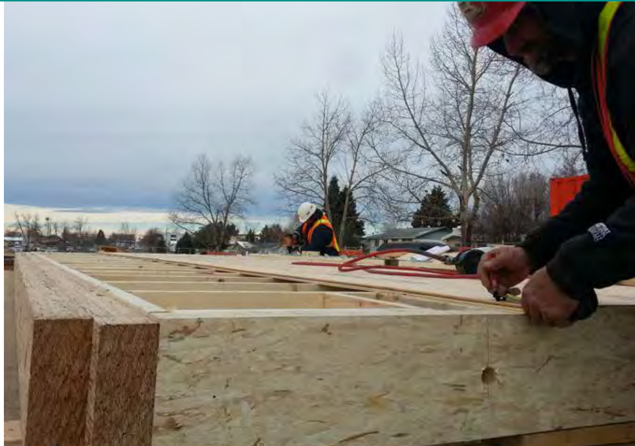
FIGURE 4.2 – HILLCREST VILLAGE: ON-SITE PREFABRICATION OF FLOOR PANELS
