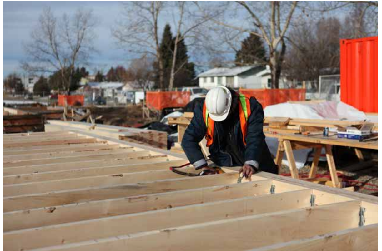
FIGURE 7.2 – HILLCREST VILLAGE: SITE PREFABRICATION OF FLOOR PANELS
