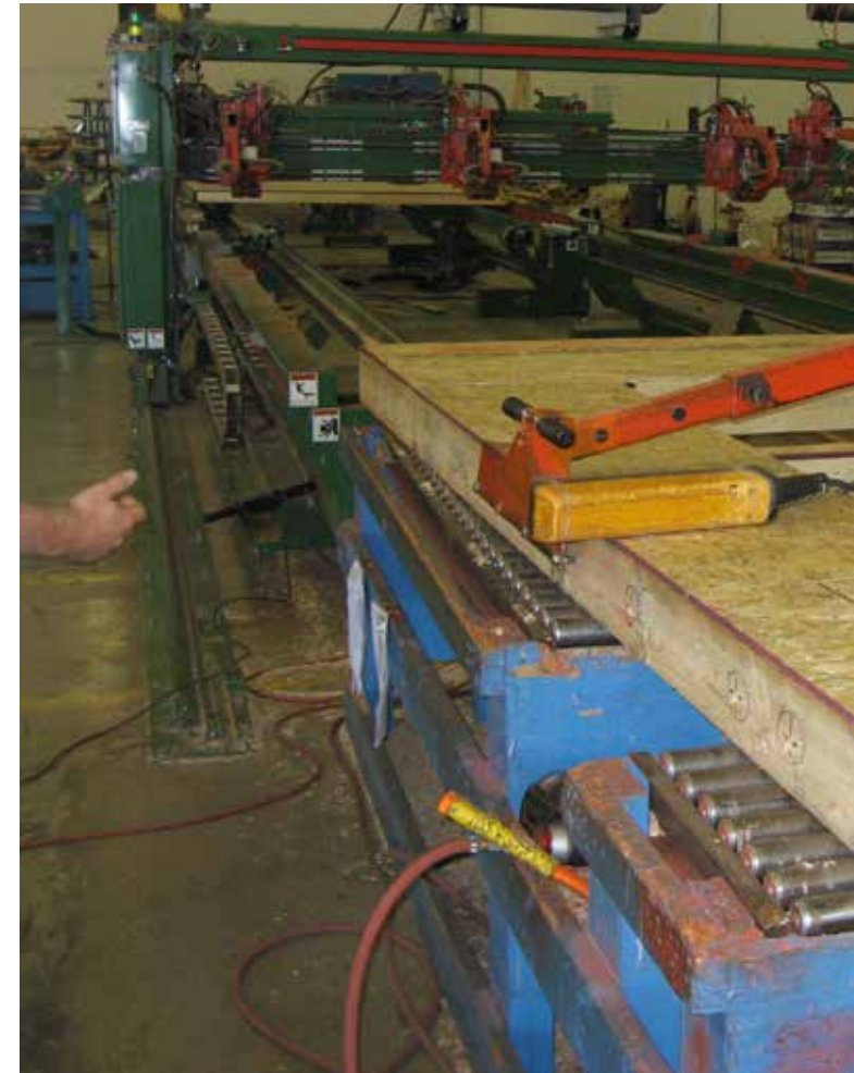
FIGURE 7.1 – HILLCREST VILLAGE: FACTORY PREFABRICATION OF WOOD-FRAME WALLS
