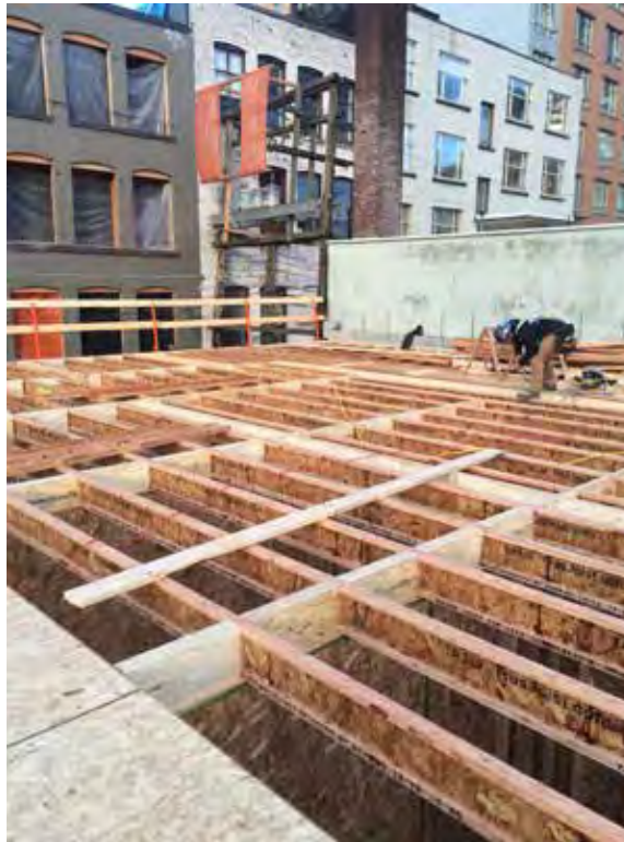
FIGURE 7.3 – SFU DOWNTOWN RESIDENCE: ALL FRAMING FOR THIS PROJECT WAS DONE ON SITE
