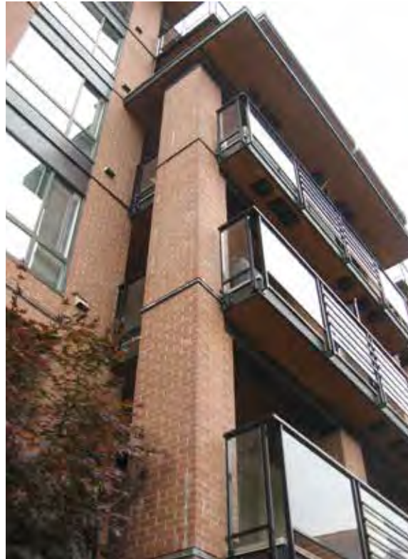
FIGURE 6.5 – THE SHORE: BALCONY SUPPORTS CLAD IN MASONRY
