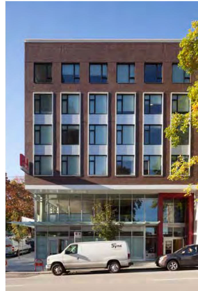
FIGURE 3.2 – SFU DOWNTOWN RESIDENCE: THE FULL-WIDTH BRICK CLADDING EXTENDS FROM THE THIRD TO THE SIXTH FLOOR
