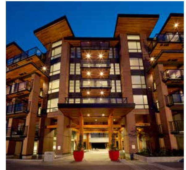
FIGURE 5.2 – THE SHORE: EXTERIOR WOOD STRUCTURES SUCH AS ENTRANCE CANOPIES, MUST BE OF HEAVY TIMBER CONSTRUCTION
