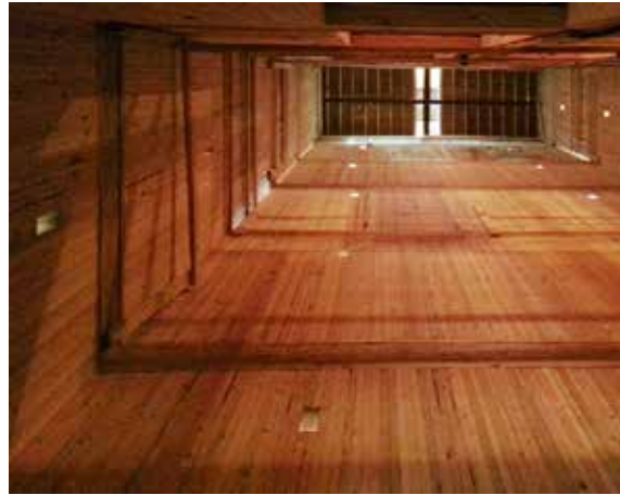
FIGURE 4.4 – HILLCREST VILLAGE: INTERIOR VIEW OF NAIL-LAMINATED TIMBER (NLT) ELEVATOR SHAFT
