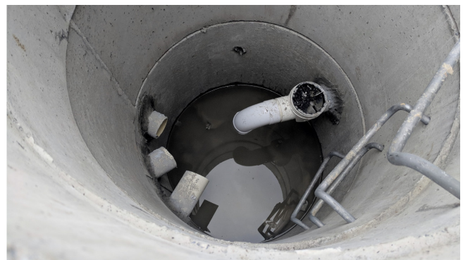
Stormwater sump. These should not be connected to any sanitary sewer
