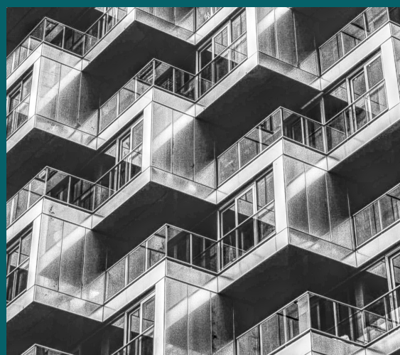
Figure 4. Roof decks can have significantly more thermal bridging compared to external balconies due to building articulation.
